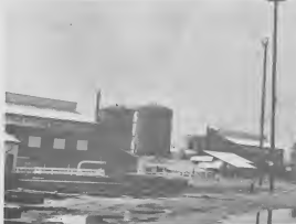
PANORAMIC VIEW of the Acid Plant reveals its sulphur plant at right, acid oil storage tanks and its two contact plants. This vital Lago operation supplies sulphuric acid necessary for alkylation and acid treating of refinery products.
